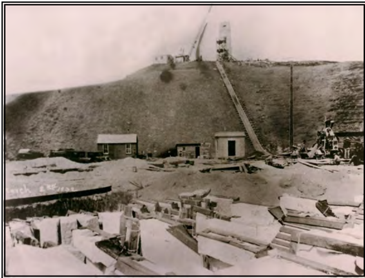
Wright Brothers Memorial Construction Circa 1930 Outer Banks History Center—David Stick Collection
