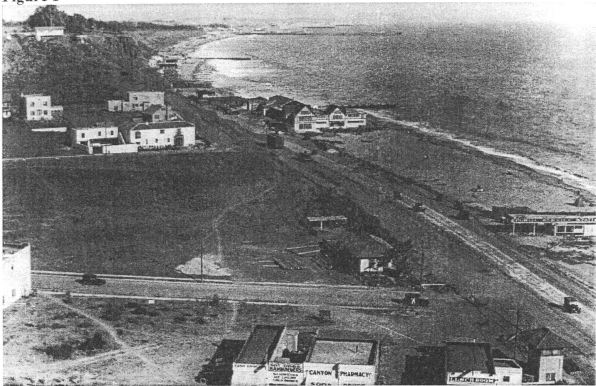
Historic photo of Bradbury House (upper left) showing entire site
